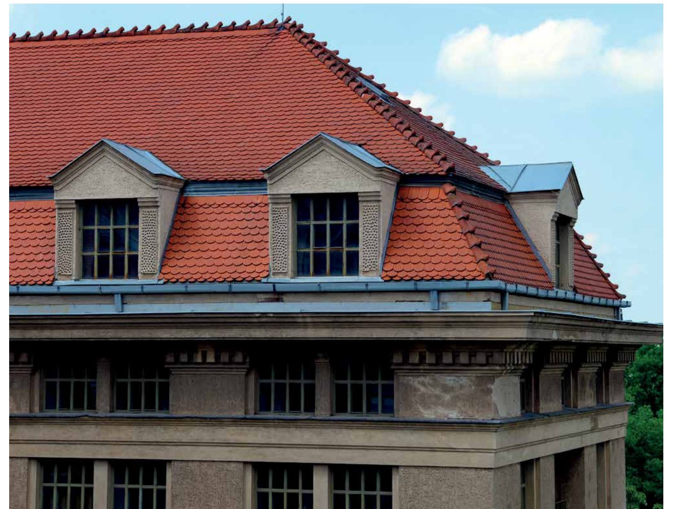
The Gutter System Used for the Rainwater Drainage of the Main Building
