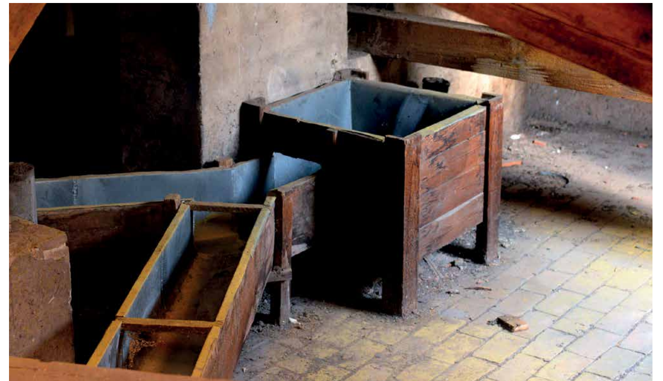
Rainwater Drainage in the Main Building
